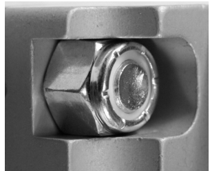
fig. 21: Bolt protrudes just beyond flush
